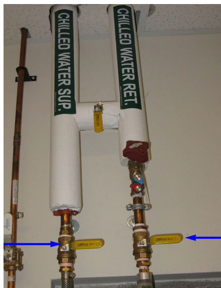
Figure 5. Chilled Water Supply and Chilled Water Return. Verify valve position (closed) in the Equipment Room
